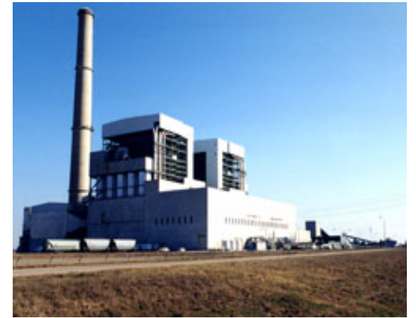
Northeastern Plant - Oologah, OK
